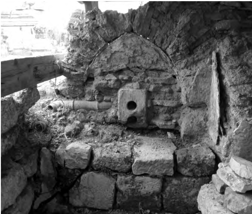
Figure 10.5 Bustān al-Khān (Baalbek): Angle of piping
